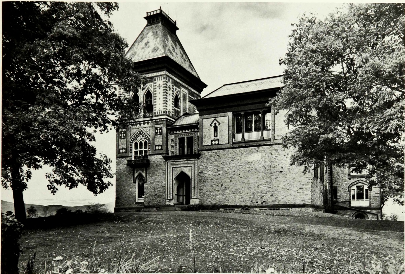
93. Olana, east façade, 1870-1872. Photo Wayne Andrews.
