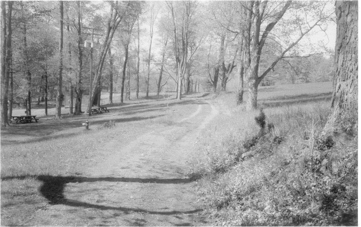
Figure 101 - Photograph of driveway to Cosy Cottage from the east, 1996.
