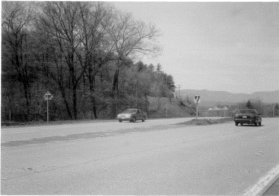
Figure 113 - Photograph of modern Route 23 as it crosses Olana, looking west, 1996.
