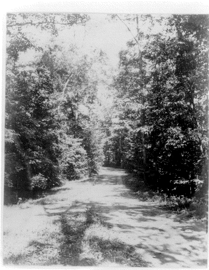
Figure 41 - Photograph of the North Road from the south, 1906.
