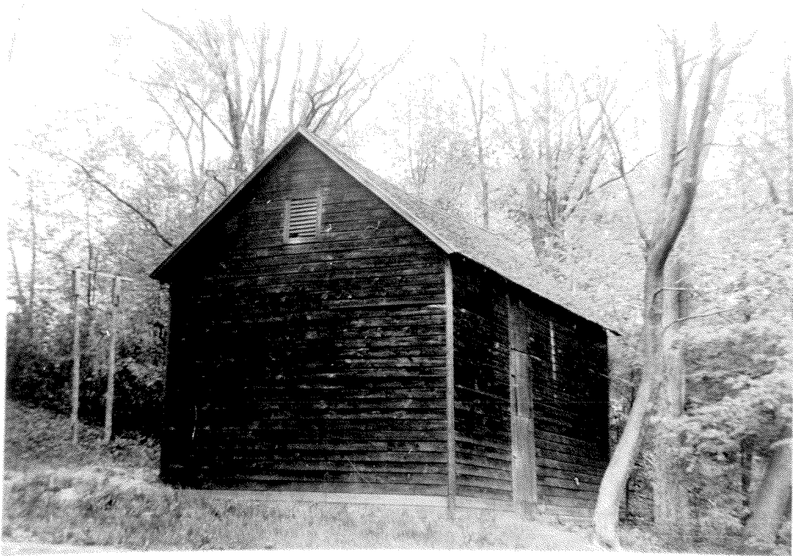
Figure 65 - Photograph of Ice House from the south, 1934.
