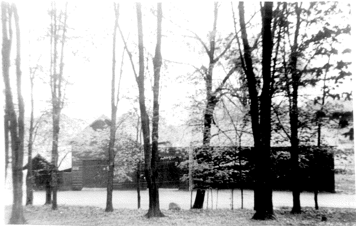
Figure 61 - Photograph of tool house, farm Stable and wagon house from the north, 1934.
