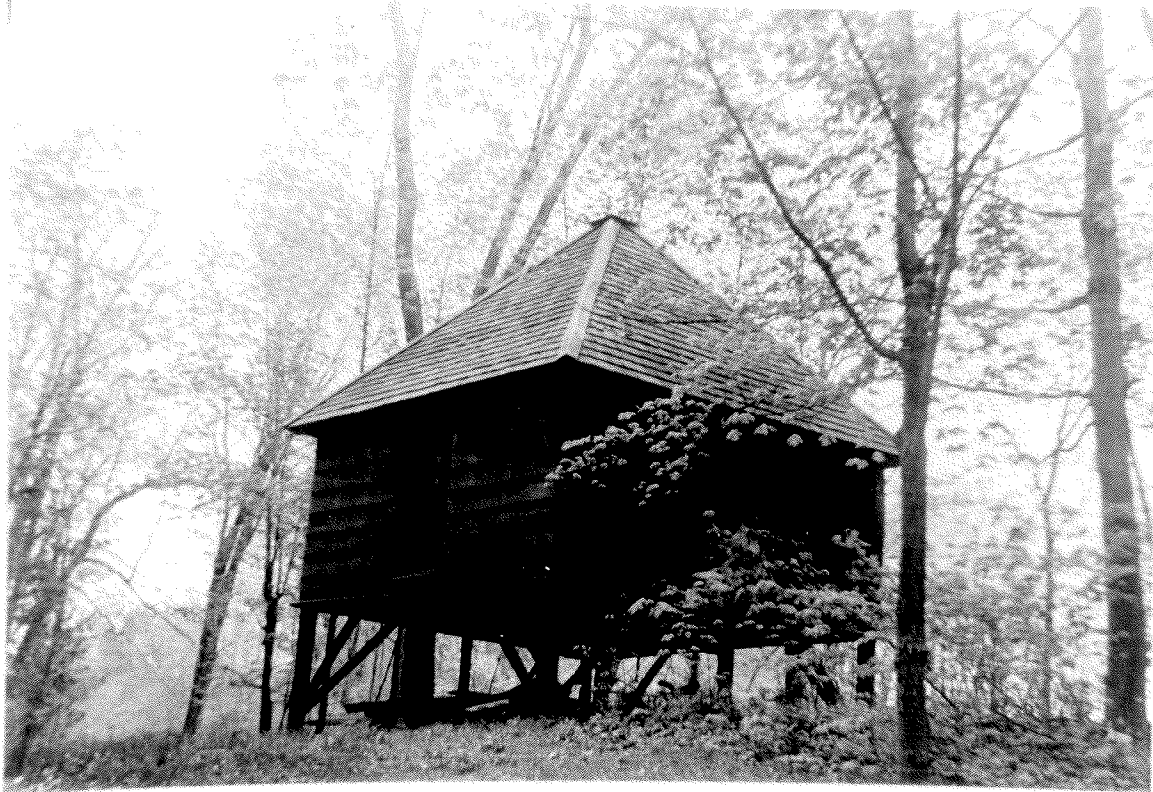
Figure 64 - Photograph of Corn Crib from the southeast, 1934.
