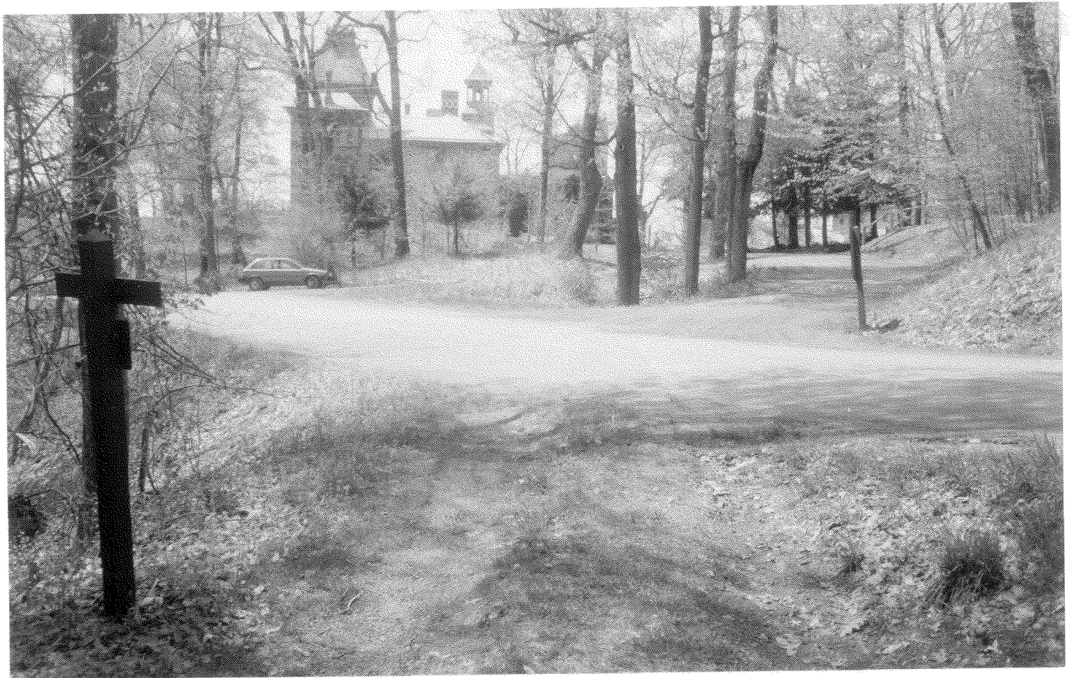
Figure 84 - Photograph of North Road approach from the north, 1996.
